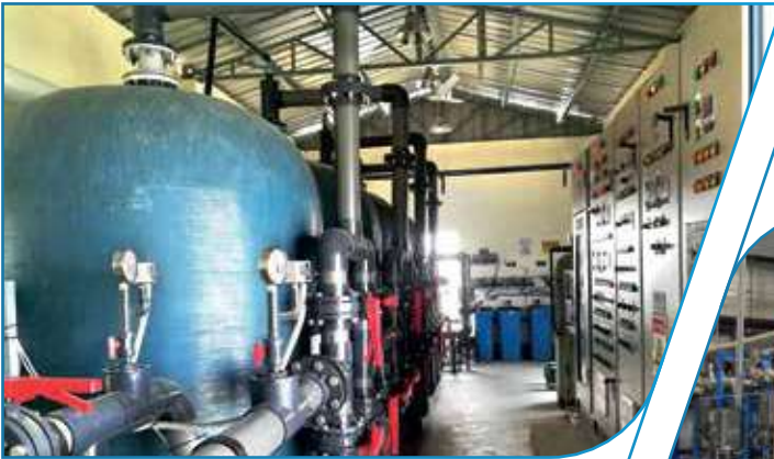
Maitree Super Thermal Power Project, Rampal Construction Water Treatment Plant: 20 m 3 /h Portable Water Treatment Plant: 01 m 3 /h
