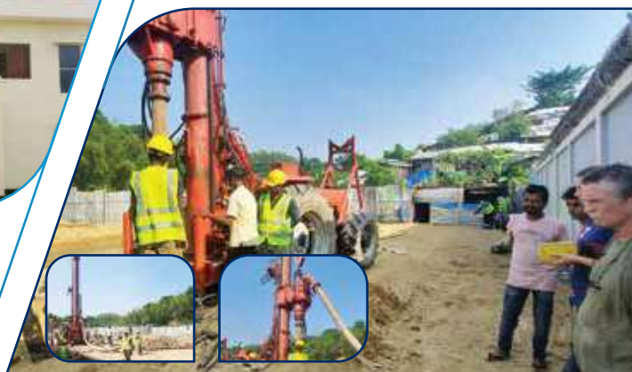
Drilling of Production Boreholes Client: Oxfam
