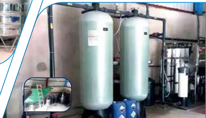
Reverse Osmosis Jar Water Treatment Plant Client: Bikrampur Drinking Water, Muktapur, Munshiganj Capacity: 02 m 3 /hr
