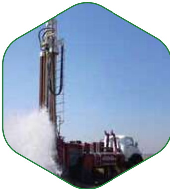
Water Wells Drilling Service
