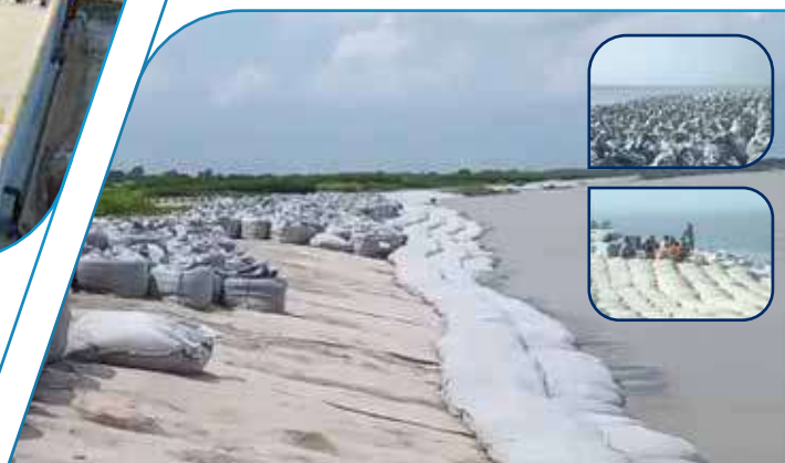
Emergency Temporary Protective Work Client: Bangladesh Water Development Board
