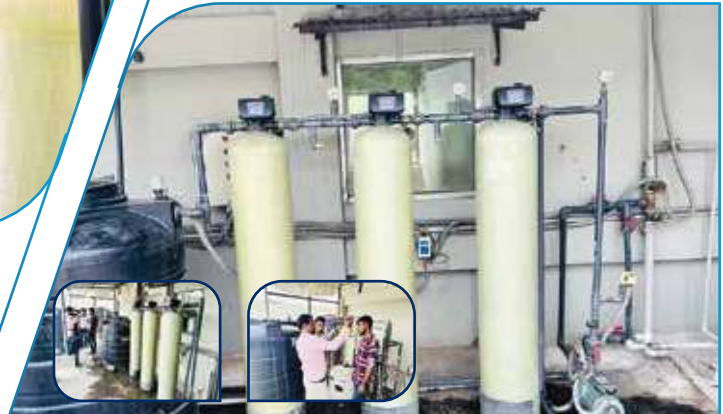
RO Plant In Roppur Nuclear Plant
